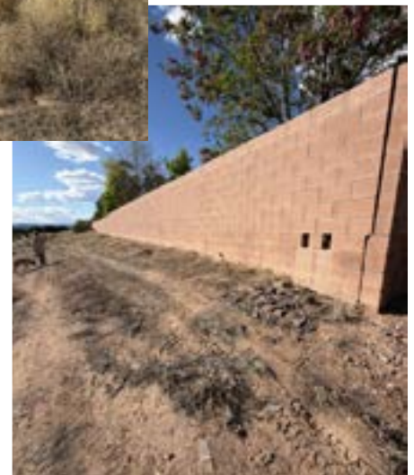
Via Punto Nuevo (backside) After Cleanup
